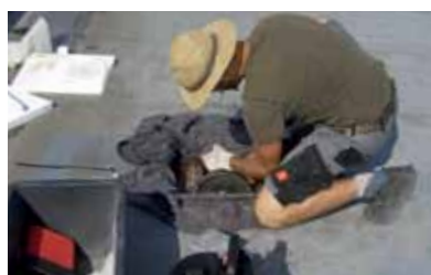
❶ Opening of the roof cladding
